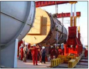
The V-94 combustion gas turbine is being installed at a substation in Kirkuk; combined with a V-64 unit, this will add 325 MW to the national electric grid.
