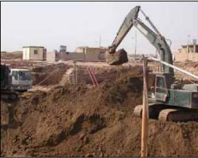
Excavation work prior to pump station construction is part of a program to restore a sewer system in a Baghdad neighborhood.
