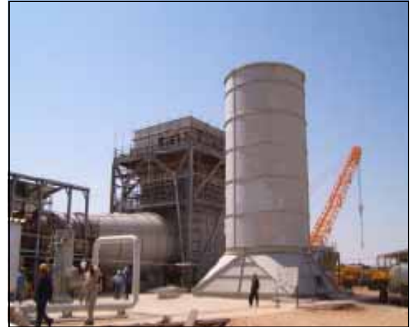
Combustion turbine and exhaust stack at the Taza substation in Kirkuk
