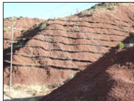
Erosion of Iraq's topsoil causes prime crop and grazing land to become barren. Terraced layers and live wattle fences have proven effective in preserving topsoil.
