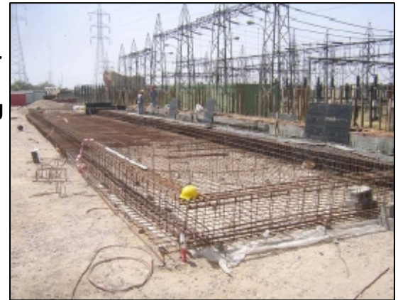
Foundation Installation for a Rehabilitated Substation
