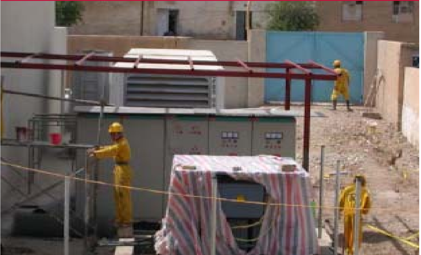
Repairs to a water treatment plant in Diyala governorate will supply potable water to 60,000 residents.
