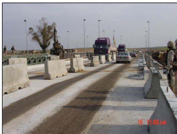
The south span of the Khazir bridge reopened for two-way traffic on January 16.
