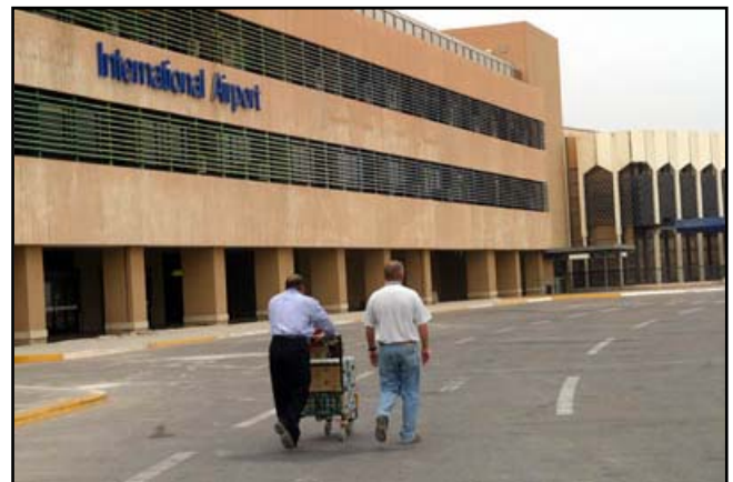
Baghdad International Airport has been refurbished and repaired with assistance from USAID and CPA. Photo: Thomas Hartwell
