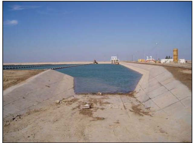
The newly restored west settling-reservoir of the Sweet Water Canal.
