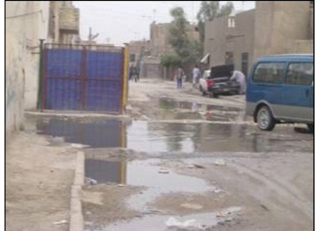
Baghdad city street covered in sludge. The Community Action Program worked with the local community to clean its streets and repair sewers.
