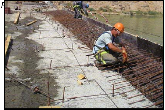
Rebar and shoring work on the Tikrit Bridge
