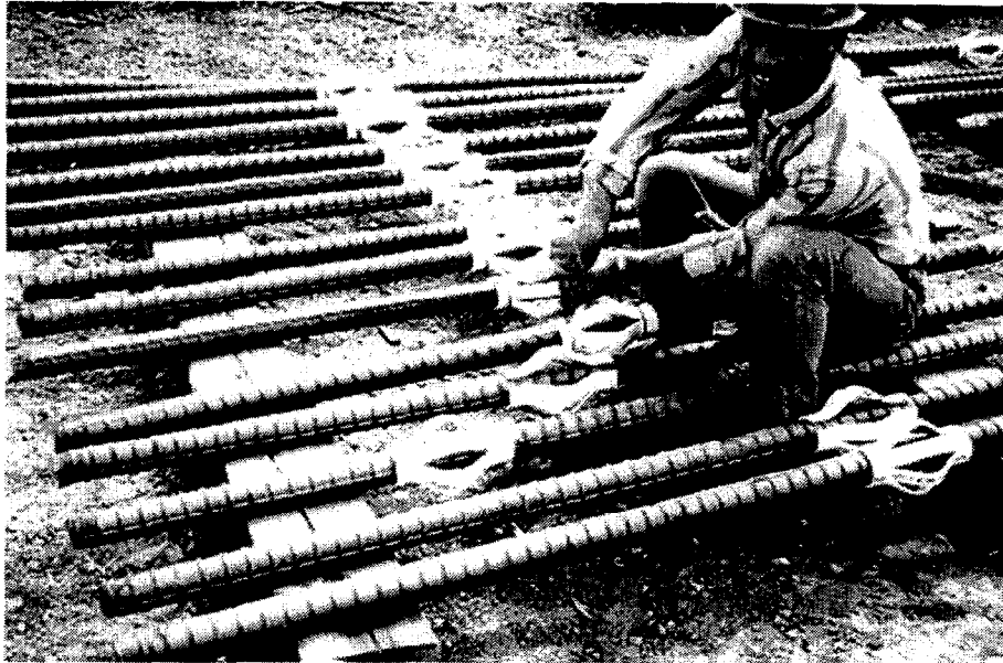
Photograph 8 - 5. Reinforcement Centralizers
