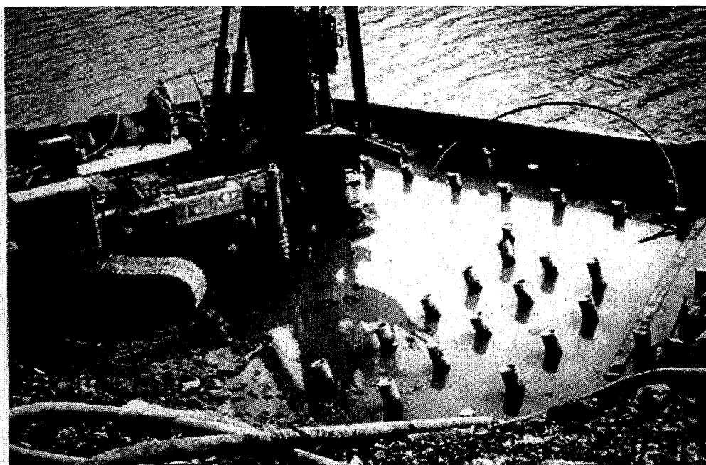
Photograph 3 - 1. 175mm Micropiles used under new abutments for bridge over Mahoning Creek, Armstrong County, PA (Pearlman and Wolosick, 1992).
