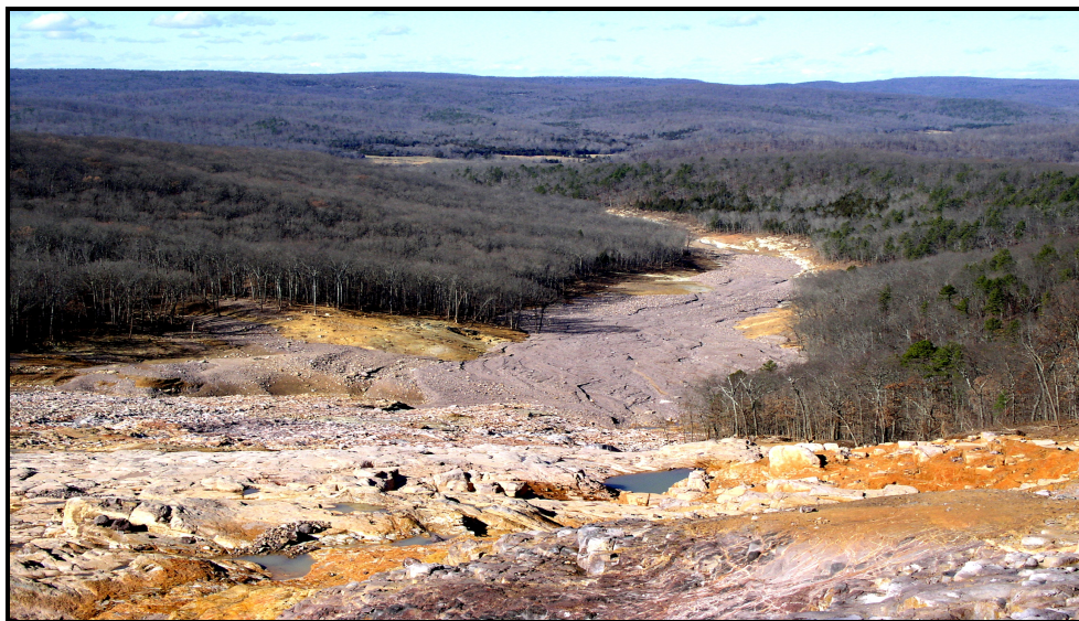
FIG. 2. Sedimentation and flow path looking northwest from breach location. (photo courtesy of D. Hoffman, 2005).
