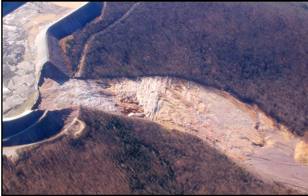
FIG. 1. The upper reservoir breach and a portion of the flow path (photo courtesy of J. Spooner, 2005)
