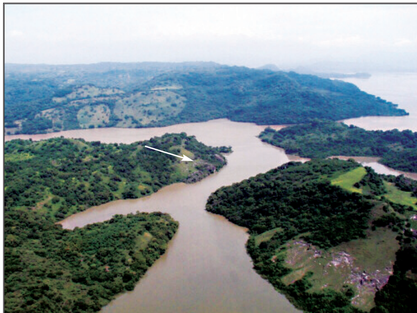
Figure 17. Shallow landslide on the shore of Embalse 15 de Septiembre. The scar was largely vegetated when this photograph was taken in September 2001.
