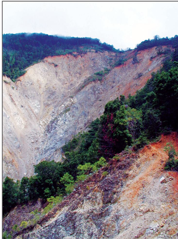
Figure 5. View to the northeast of the upper part of El Zompopera landslide. The collapse of unstable blocks in the upper part of the landslide destroyed a road at the crest of the ridge. Many unstable blocks remain in the upper part of the slide and a catastrophic collapse of those blocks could potentially dam the Río La Palma at the bottom of the valley.
