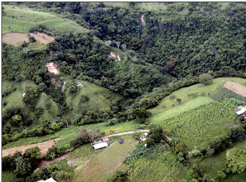
Figure 12. Scars of landslides caused by the 13 February 2001 earthquake west of San Lorenzo. Like the Hurricane Mitch landslides, these shallow landslides caused little serious damage, but repeated sliding here shows that these slopes are highly susceptible to landslides.
