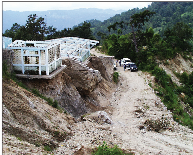
Figure 6. View of the El Pinar landslide and the abandoned school. A new road has been graded across the head of the landslide, which slid into the valley of the Río La Palma o Las Pozos on the right. Future movements on the landslide will likely disrupt the new road.
