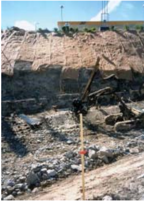
Figure 5. Hollow, drilled-in soil nails are used to stabilize a slope.
