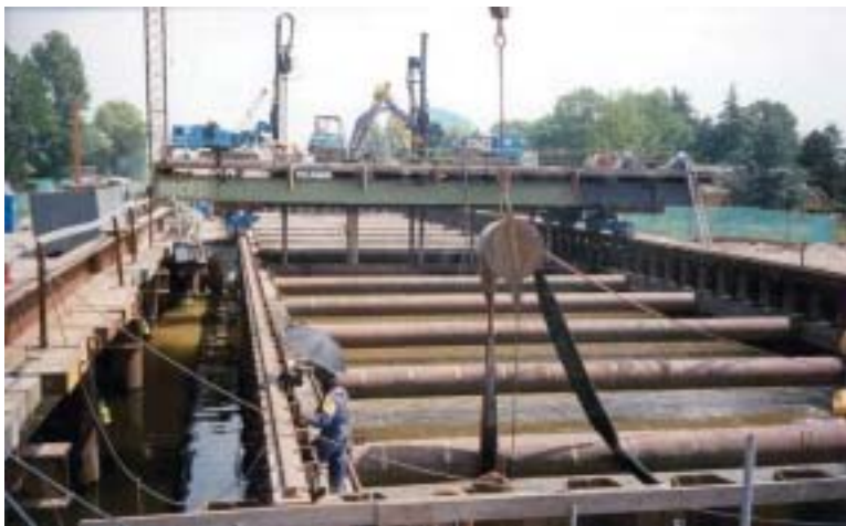
Figure 10. Site visit to the Betuwe railway line (in the Netherlands).
