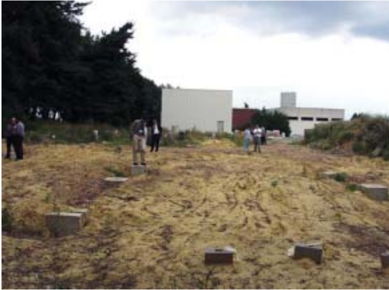
Figure 20. Screw pile test site at the Belgian Building Research Institute (BBRI).
