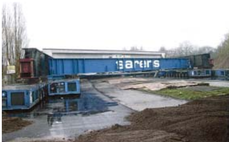
Figure 1. Example of rapid bridge replacement showing transport of new bridge with specialized lift (from Belgian presentation).
