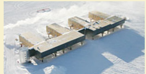
Aerial view of the new elevated building at Amudsen-Scott South Pole Station. The silver cylindrical structure on the left houses a staircase. The two main sections of the building contain the dining facility, science labs and office space. The four wings contain dorm rooms, laundry facilities and a gymnasium. A dedication ceremony for the new building will be held January 12, 2008. Credit: Robert Schwarz, NSF
