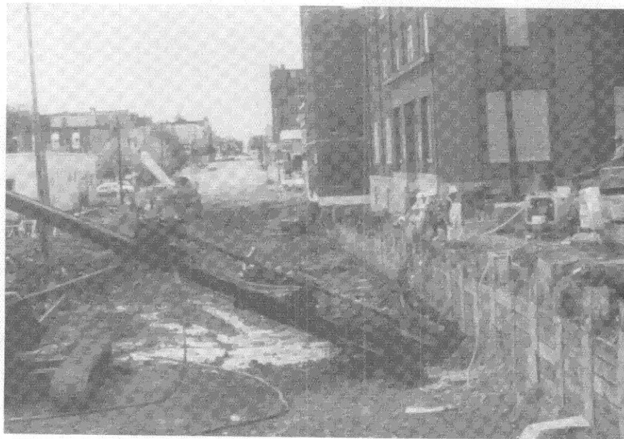
Figures 8D and 8E.--Anchor Drilling
