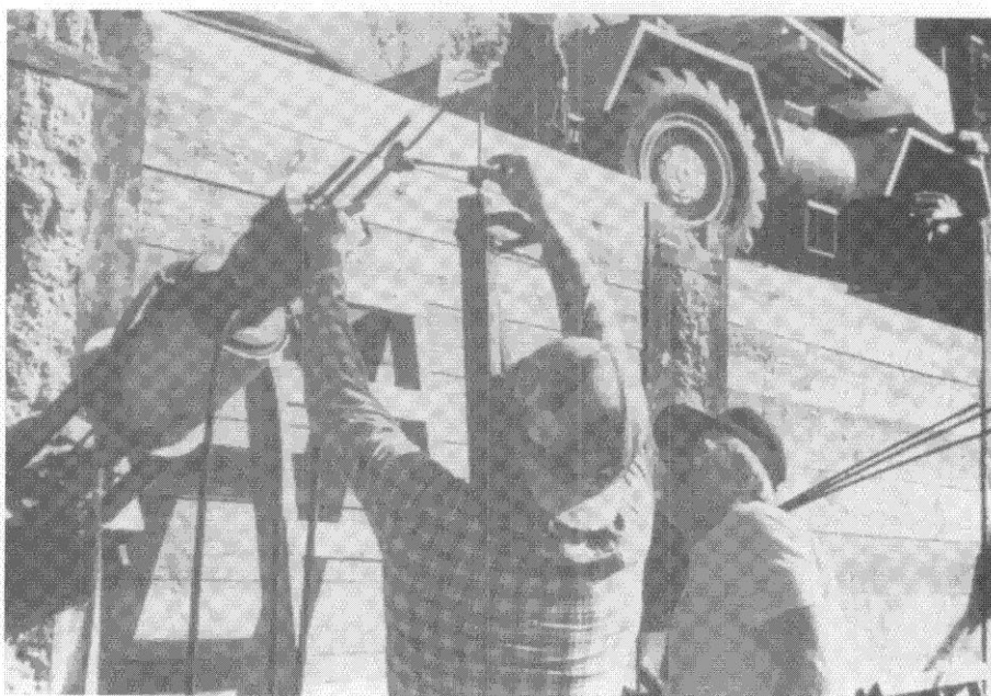
3A.--Testing of First Anchor Row
