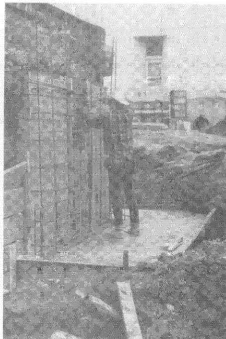
Figures 8A, 8B, and 8C.--Building Underpinning Operations
