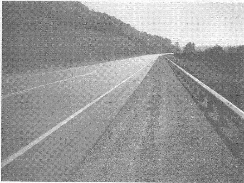
Figure 6A Embankment Stable With No Evidence of Movement 3 Years After Construction
