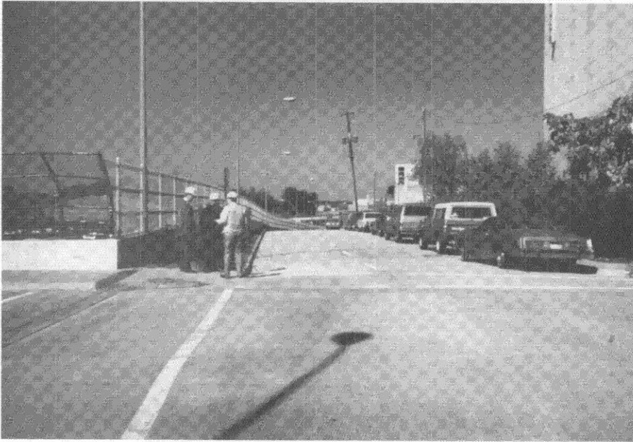
3E.--Stable Roadway, 1988 Above Wall - No Pavement Cracks
