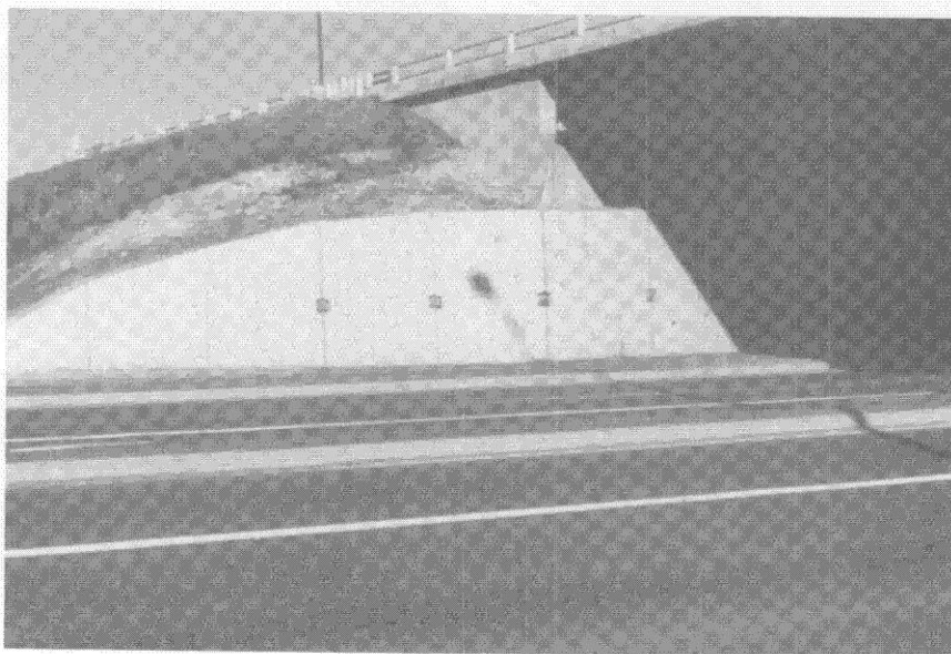
Completed Dimond Boulevard Wall
