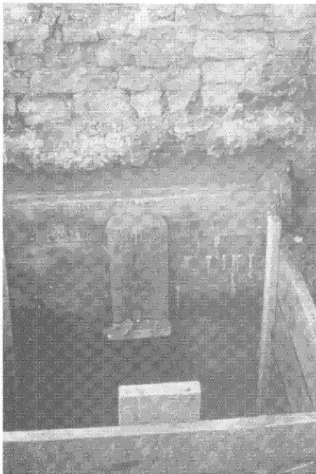
Figures 8A, 8B, and 8C.--Building Underpinning Operations
