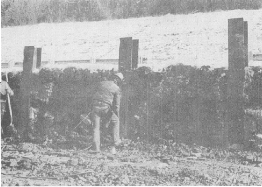
Figure 8. Piling in Place and Excavation of Embankment.
