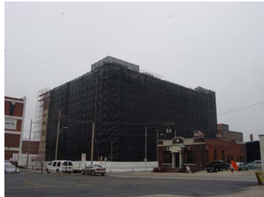
Figure 2 PCB Treatment Building with Scaffolding and Scrim
