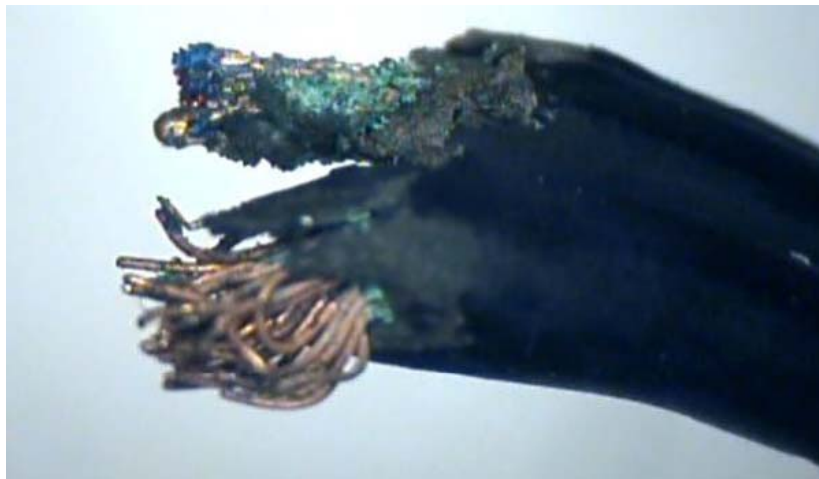
Figure 7. Close-up of Wiring to the Fourth Socket
