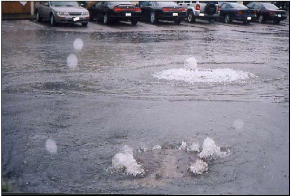
Two overflowing manholes flooding a street and parking lot in Rhode Island with contaminated water.
