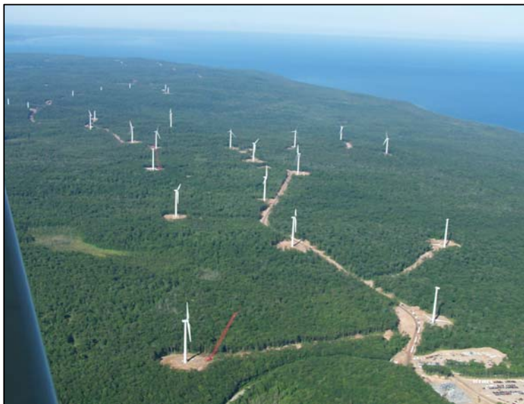
Figure 4-8. Brookfield Power completed Prince Wind Energy Project in 2006. It is the largest wind farm in Canada. Photo credit: Gary Stewart, OMNR.
