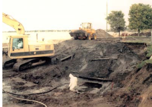
Coal tar removal at Clear Lake Coal Gas, Clear Lake, Iowa 1994
