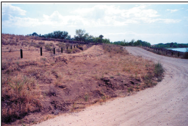
Damage from illegal off-road driving at Gotts Point.
