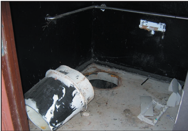
August 2006 damage to the Gotts Point outhouse.
