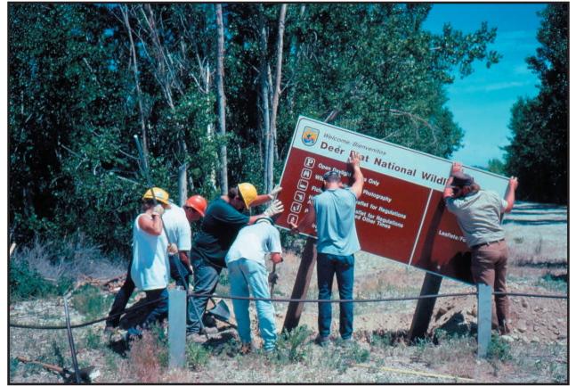
A refuge YCC crew installing a regulation sign.
