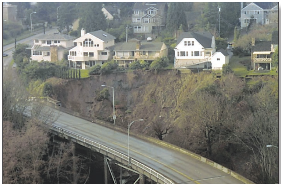
These houses overlook the Magnolia Bridge area of Seattle. The white house on the right side hangs precariously over the headscarp of a large landslide (photo by Hugh Shipman, Washington Department of Ecology).
