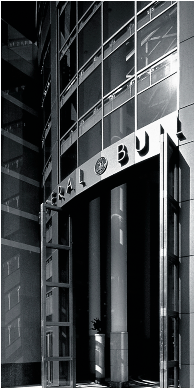
Oakland Federal Building, Oakland, CA.
