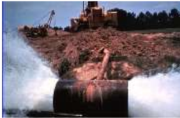
Figure III-3. Blowing Down a Pipeline After Hydrostatic Testing
