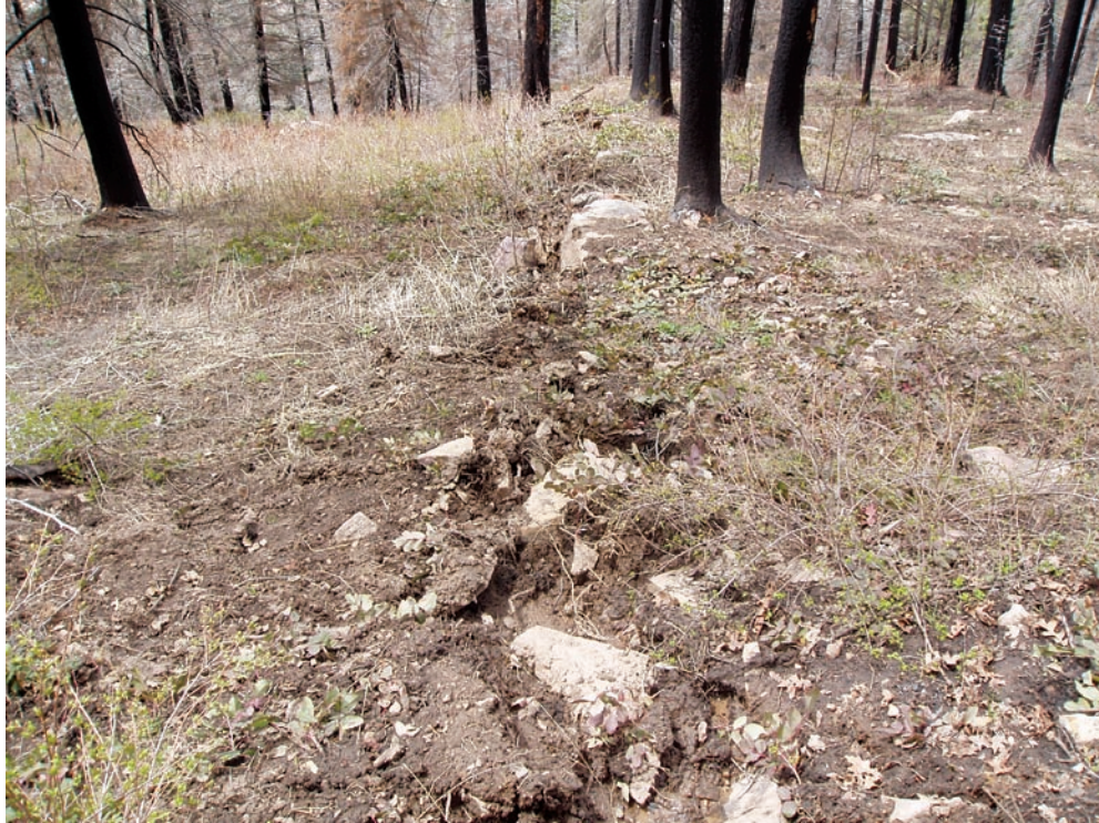
Figure 9. Lateral shear zone along the margin of a translational landslide that was active during spring 2005 within the Florida River landslide complex. Landslide is on the right side of the ground fracture. Trees along shear zone are about 0.3 m in diameter.
