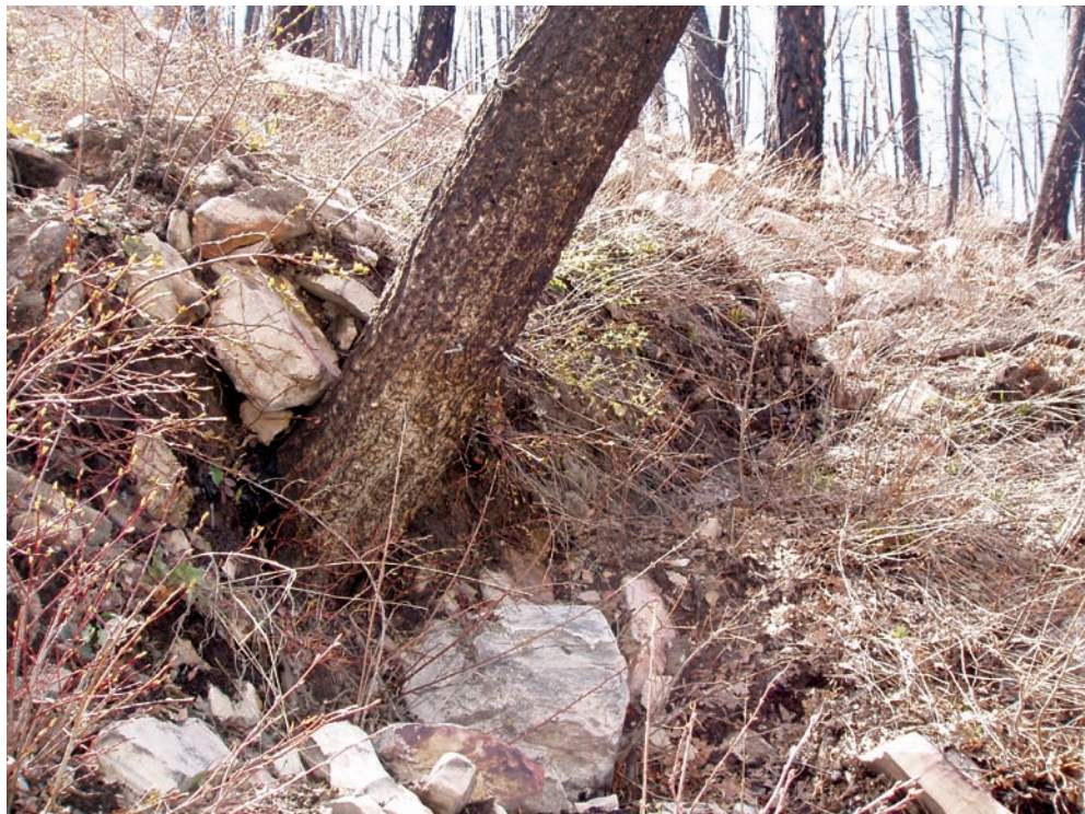
Figure 10. Toe of a translational landslide that was active during spring 2005 within the Florida River landslide complex. The toe is thrusting over the leaning tree that is about 0.4 m in diameter.
