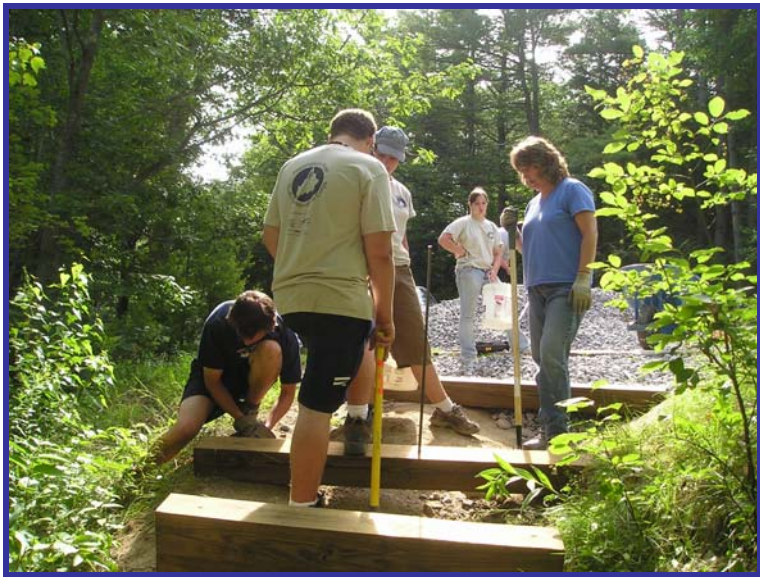
Betty Williams of the Cumberland County Soil and Water Conservation District guides the Presumpscot River Youth Conservation Corps as they install infiltration steps on an eroded trail to the Presumpscot River. Credit: Lisa Vickers, Presumpscot River Youth Conservation Corps
