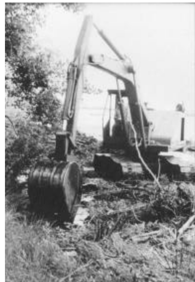
Wetland being filled
