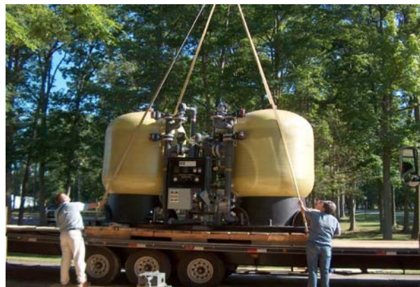
Queen Anne County's new arsenic water treatment equipment
