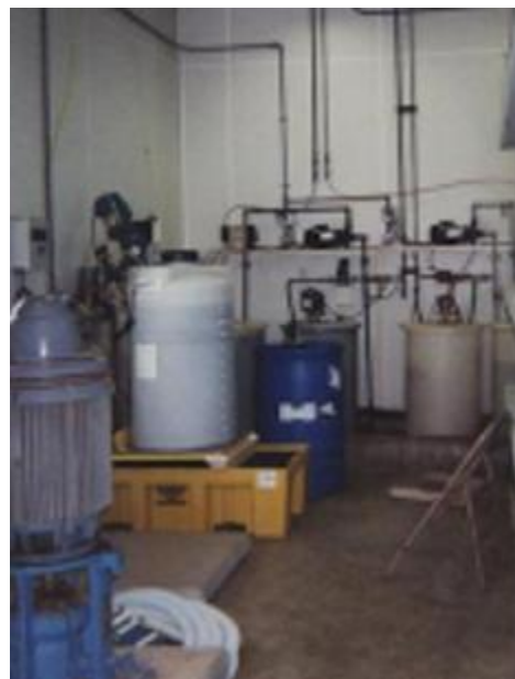
Lidgerwood's new arsenic water treatment equipment
