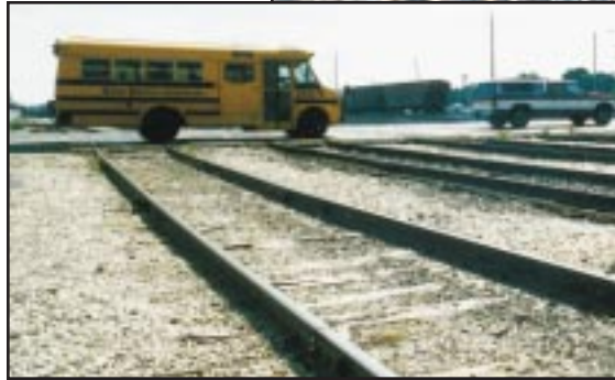
At-grade railroad crossings present a host of safety and routing concerns.
