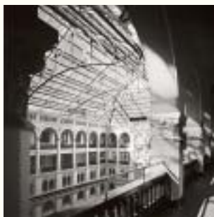
NANCY HANKS CENTER OLD POST OFFICE BUILDING WASHINGTON, DC 1892-1899 WILLOUGHBY J. EDBROOKE
