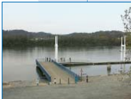
Chattanooga's floating dock will include artistic lighting in response to public input.
