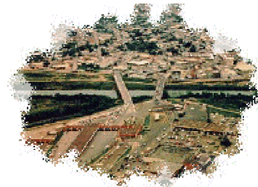
International bridge near McAllen
