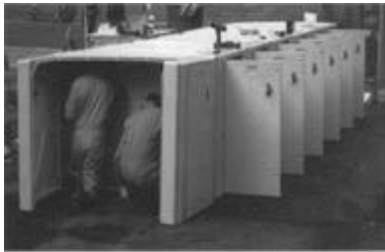
Installing bicycle lockers
