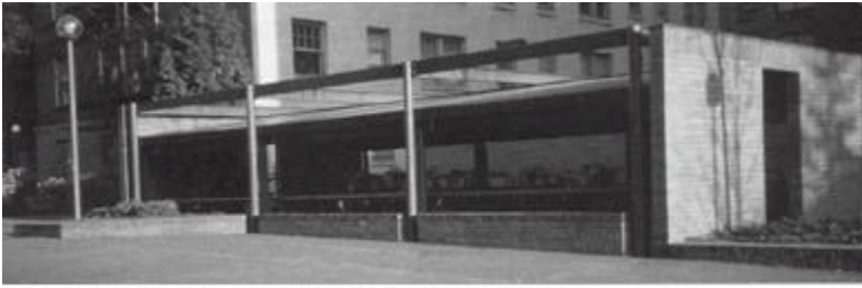
Covered parking at Portland State University
