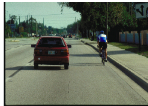
Figure 2. Typical wide curb lane.
