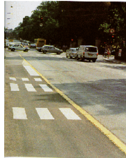
Figure 5. Profiled marking at a bus stop to separate bicyclists from bus passengers. Source: Safety of Cyclists in Urban Areas, 1994
