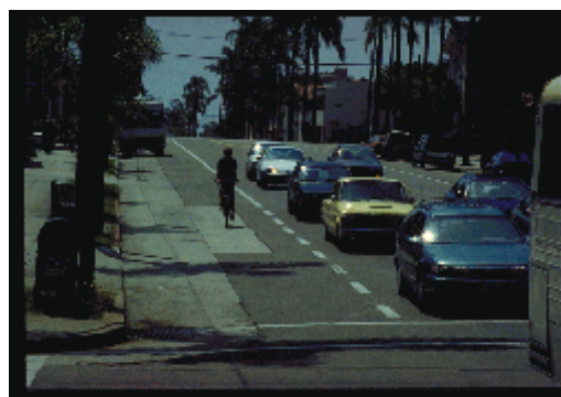
Figure 7. BL dashed to intersection.
