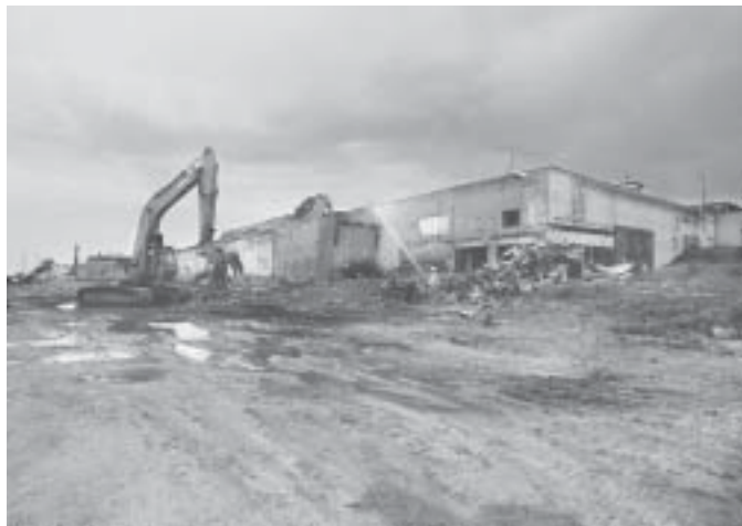
Crews work to demolish a building at Rocky Flats.
