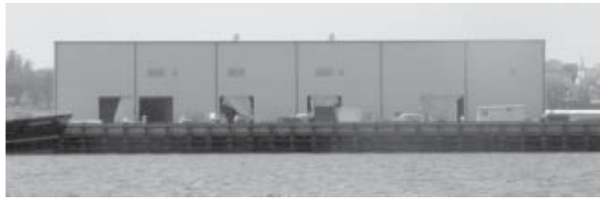
EPA's new sludge dewatering facility at New Bedford.
