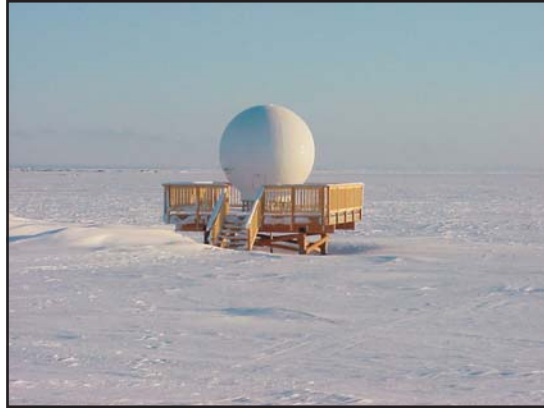
NOAA National Environmental Satellite, Data, and Information Service (NESDIS) 3-m (left) and 4-m (right) High Resolution Picture Transmission (HRPT) downlink antennas for the NOAA Polar Operational Environmental Satellite (POES) at the observatory site. These antennas allow for near-real-time downloads of ice and cloud conditions over the Arctic Ocean.
