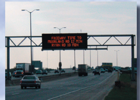
The variable message sign displays travel times. Photograph courtesy of Wisconsin DOT.
