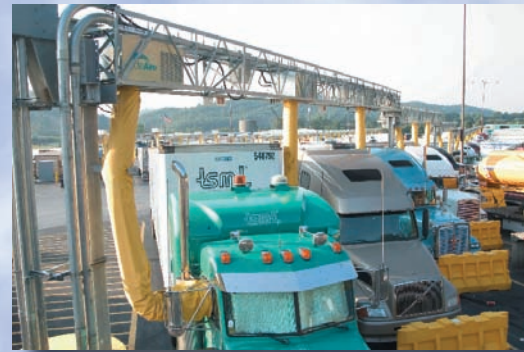
A simple window adapter makes this electrification system compatible with many models of long-haul trucks. Photograph courtesy of IdleAire.
