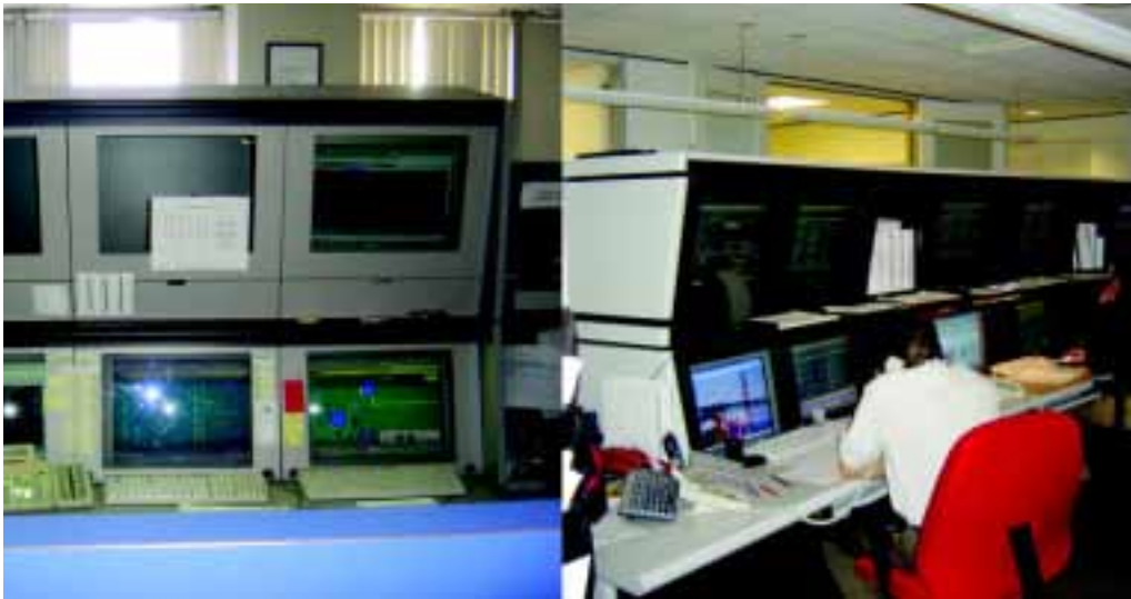
Figure 4.3. Centers with stacked monitors due to space constraints.
