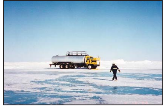
Water spray truck drawing water from a local North Slope lake. Trucks like this are used to create the ice roads.
