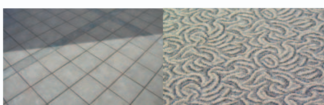
Low volatile organic compound paint, adhesives, glues, carpet, and floor tiles were used to finish the building.
