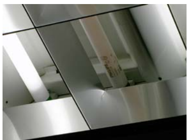
Example of a mercury fluorescent lamp on the ceiling of a classroom.
