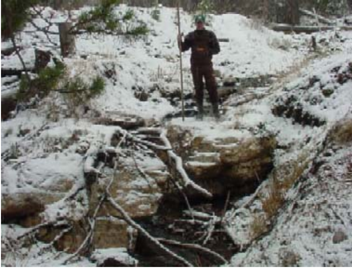
Figure 5. Fish barrier created by a poorly designed road closure.
