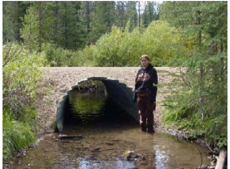
Figure 22. Some culverts such as the one on the left in Garden Creek can completely block upstream fish passage whereas other culverts such as the one on the right in Mill Creek do not interfere with fish passage.
