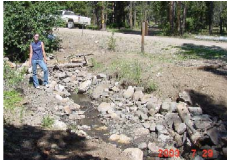
Figure 8. Newly constructed stream channel (same area shown in Figure 6).
