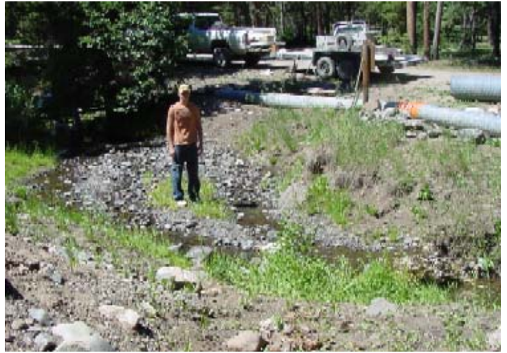
Figure 6. Degraded stream channel created by a poorly designed road closure.
