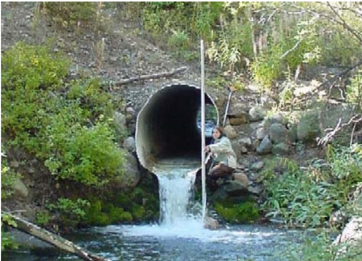
Figure 22. Some culverts such as the one on the left in Garden Creek can completely block upstream fish passage whereas other culverts such as the one on the right in Mill Creek do not interfere with fish passage.
