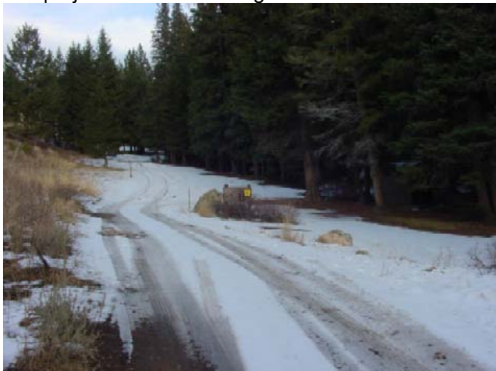
Figure 11. Mill Creek Trailhead in 2001 prior to restoration.
