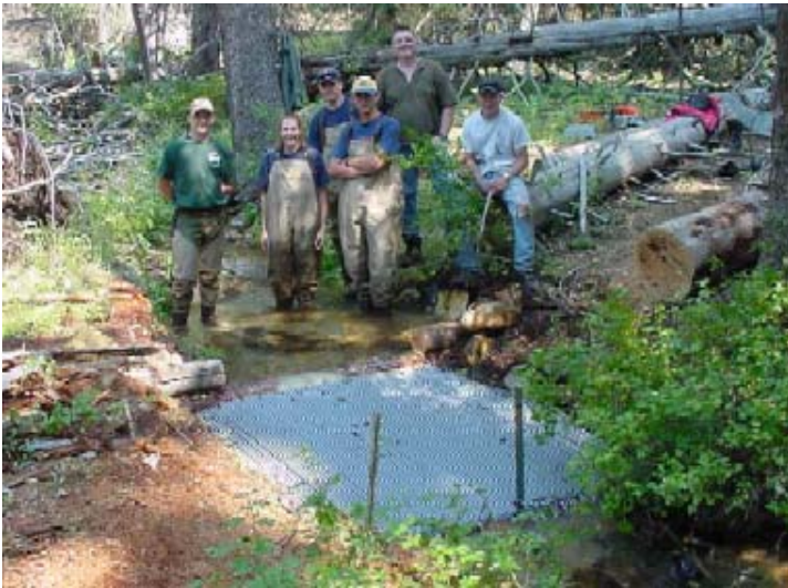
Figure 9. Squaw Creek fish barrier that was installed in 2001 to prevent brook trout from reinvading the treatment area.
