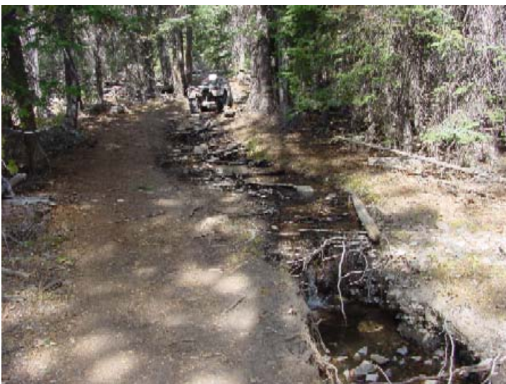
Figure 20. Stream erosion in Timber Creek associated with a poorly located OHV trail.
