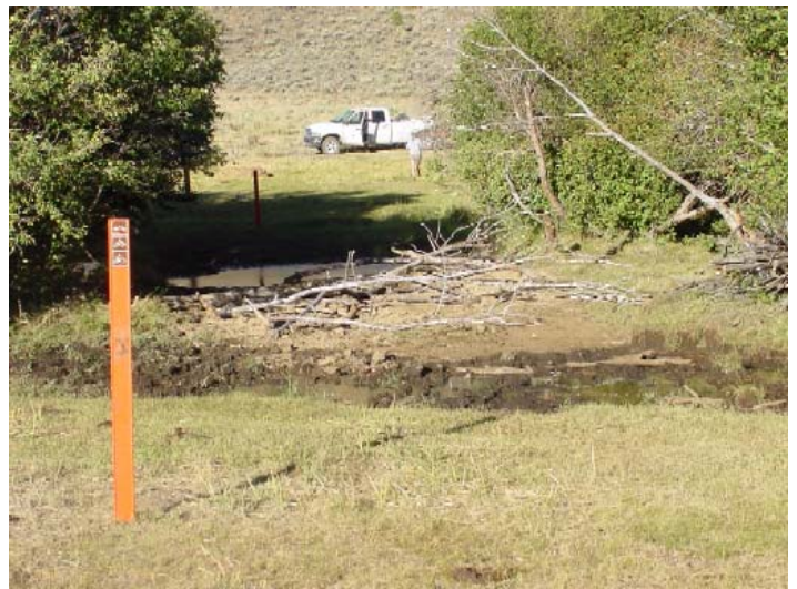
Figure 32. Damaged area following the completion of the restoration project.
