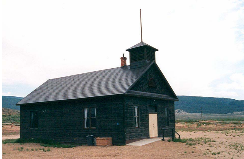
Figure 14. Lodore School Building
