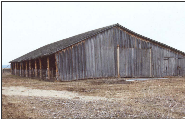
Figure 3. Long Barn at the Historic Sod Ranch
