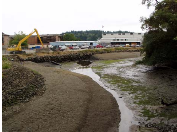
Construction of the Additional Tidal Barrier
