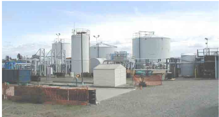
EPA plans design changes in Wyckoff's cleanup plant.
