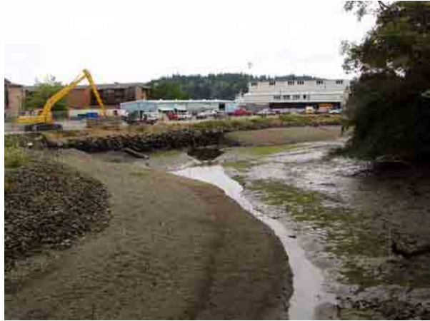
Construction of the Additional Tidal Barrier
