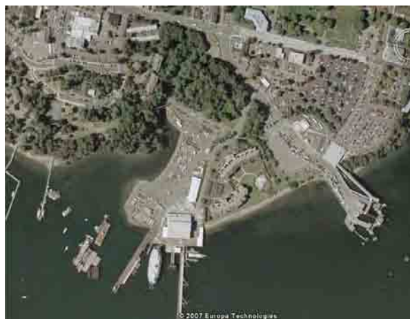
Aerial View of the West Harbor (Operable Unit 3)
