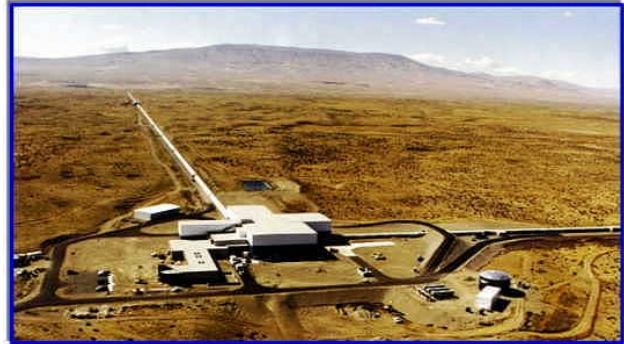
FIG. 9. The Hanford Observatory, one of LIGO's two laser interferometers for detecting gravitational waves.
