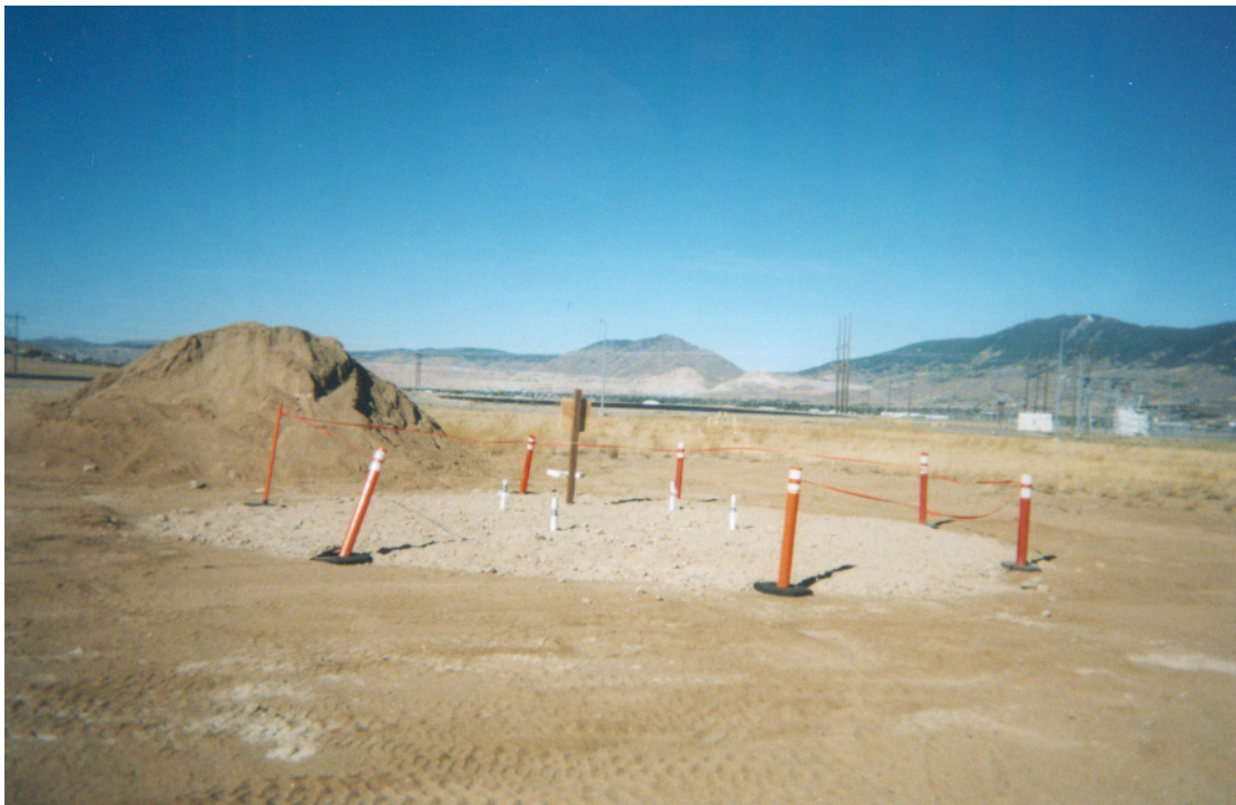
Figure 4-6. Test cell final configuration September 30, 2003.
