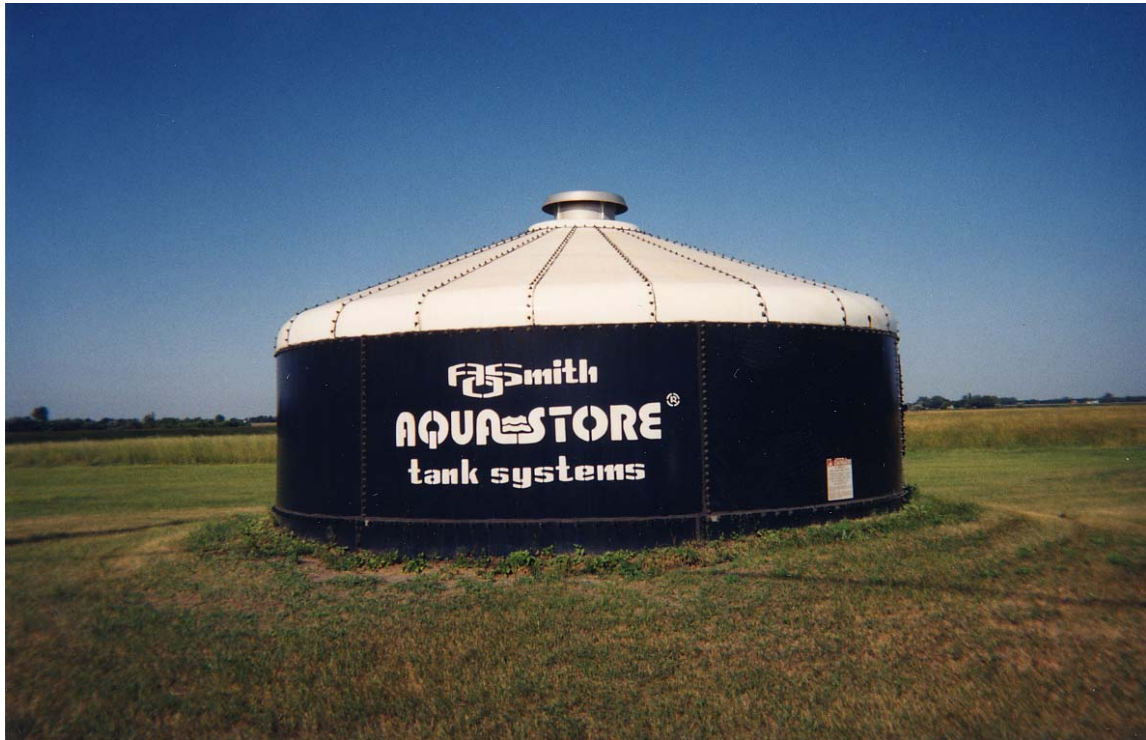
Figure 4-3. Pre-Existing Backwash Sludge Holding Tank
