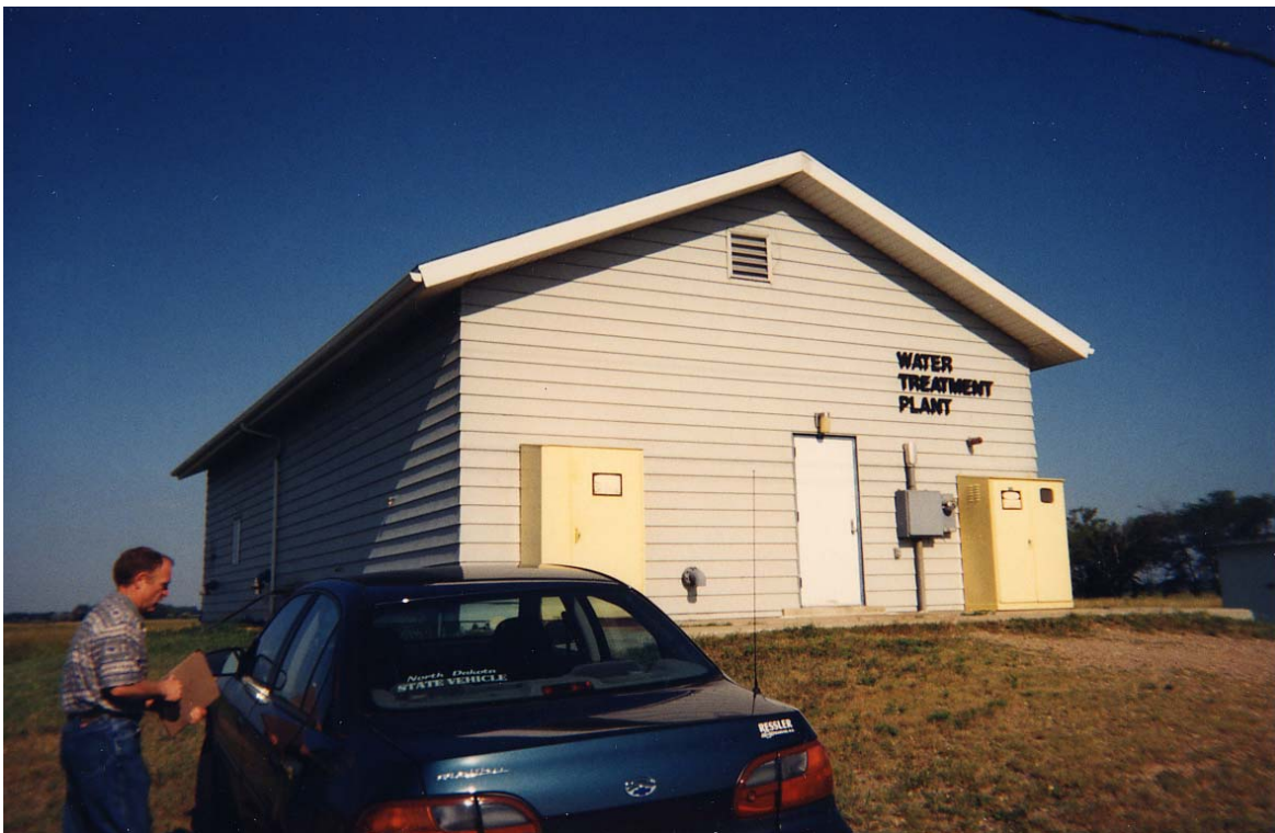
Figure 4-1. Pre-Existing Water Treatment Facility at Lidgerwood, ND
