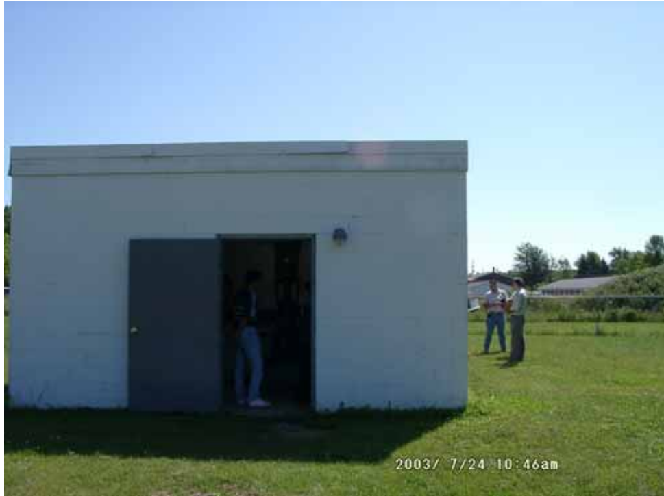
Figure 4-2. Former Pump House at Brown City, MI, Site
