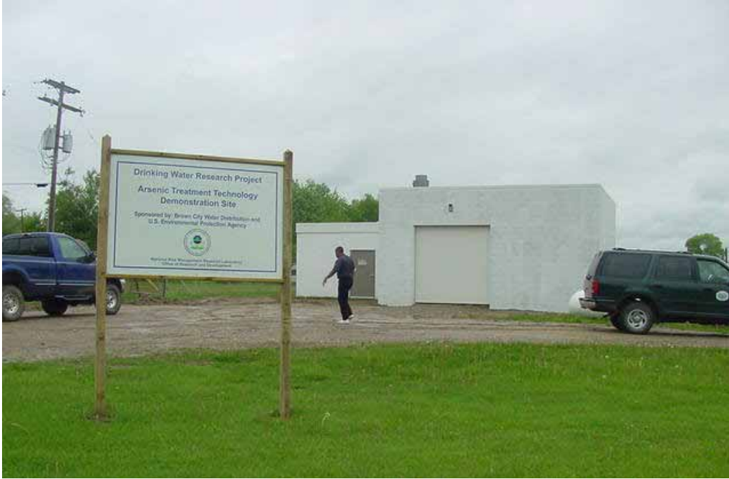
Figure 4-7. New Building at Brown City Adjacent to the Pre-Existing Pump House (on the left)
